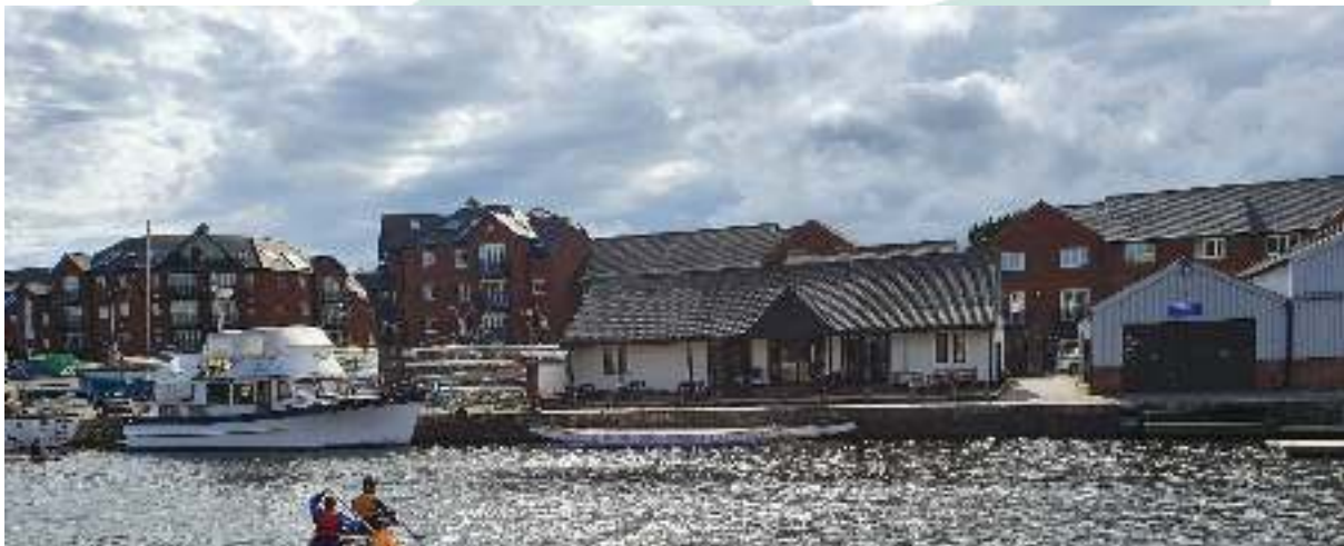
Part of the site for Exeter City Living's proposed waterside redevelopment: Exe Water Sports Association HQ (centre) with boatsheds (right) and boatyard (left)
