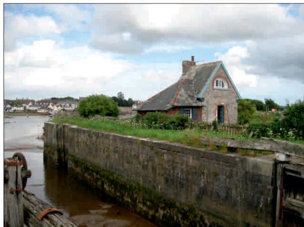
The Lock House is an attractive building of limestone with a steeply-pitched roof, having a later addition in two colours of brick.
